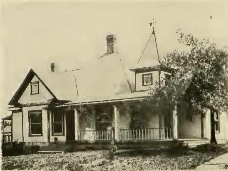
RESIDENCE OF A. W. PFEIFER. North Sixth Street.
